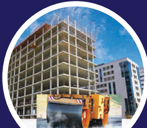
CIVIL ENGINEERING WORKS
