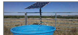
Solar pump used for live stock drinking in Australia
