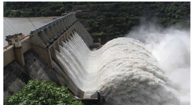
Hydro /Dam Engineering
